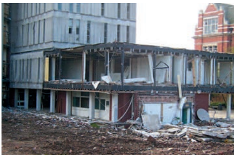
James Went Building being demolished 2007
